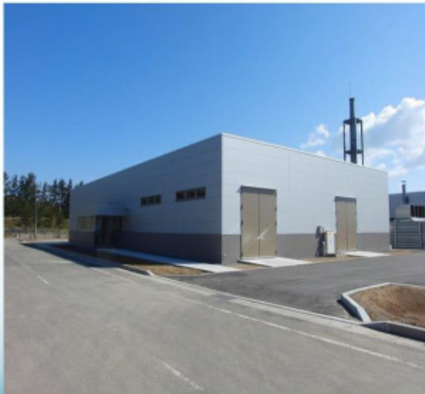
Joint Research Building
